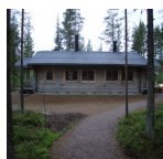
Facilities in Vasikkavuoma ( County Administration Board of Norrbotten, 2008 )
