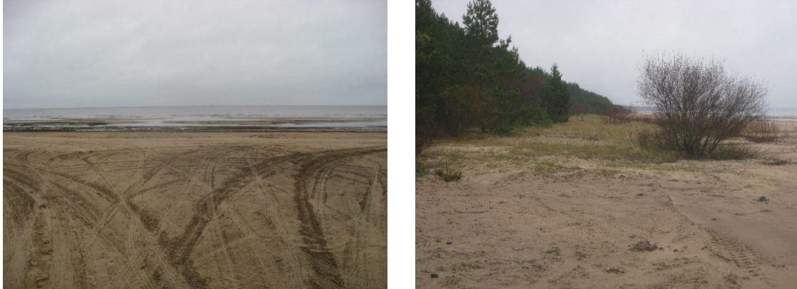
Figure 5. a) Looking westward from the construction corridor to where the breakwater was installed during pipeline installation; b) looking southward along the edge of the construction corridor showing height of foreshore dunes and vegetation.
