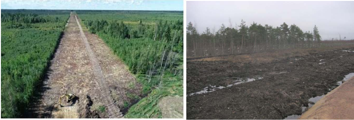
Figure 12. Working corridor of layered logs (left) and following removal (right)
